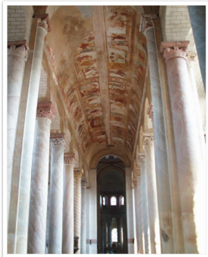
The painted barrel vault at the Abbey
