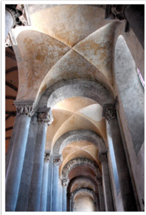
The aisle of the Abbey Church at Mozac has groin vaults supported on transverse arches.
