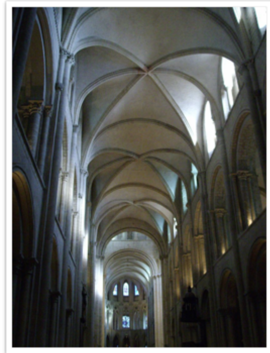
The ribbed vaults at Saint-Étienne, Caen, are sexpartite and span two bays of the nave.
