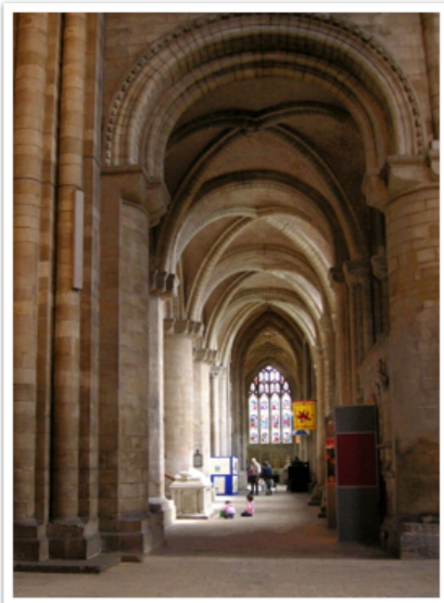
The aisles at Peterborough Cathedral have quadripartite ribbed vaults. (The nave has an ancient
