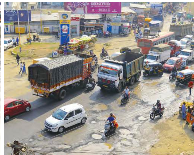
Fig. 7.27. Potholes on the roads
