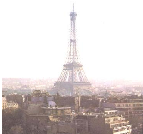
The Entrance Pavilion, Exposition Universelle 1889 • Designed by Gustav Eiffel and Maurice Koechlin • Extensive use of iron, 300m high
