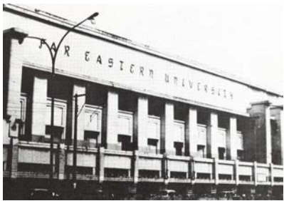
FEU Main Building • by Pablo Antonio
