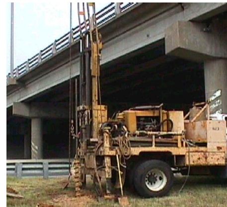
Soil Boring Rig.
